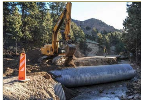
Culvert installation, Jamestown, CO, 2013. Photo credit: Michael Rieger/FEMA
